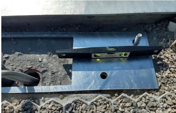
To tilt the floor plate, insert large washers below the floor plate until it becomes level.
